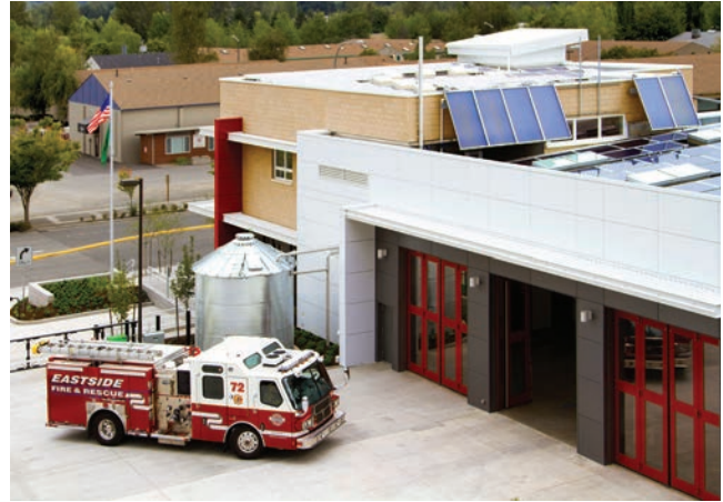
An 8,000 gallon cistern provides water for toilet flushing, laundry, irrigation, and truck washing. A 30 kW solar array reduces the station's EUI to 22.3.
