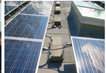
ABOVE A 30 kW solar array contributes 5 kBtu/ft 2 -yr of energy to the building.
